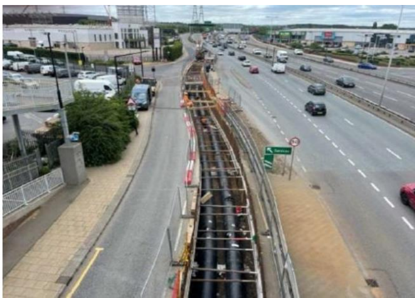
Energetik – new Energy Centre and heat network installation
