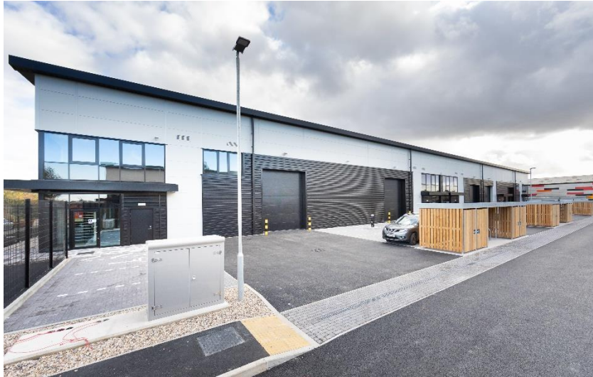
First phase of Montagu Industrial Estate regeneration programme
